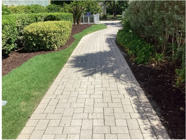
Masonry pavers at east elevation of building
