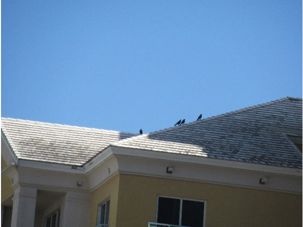
Concrete tile roof overview
