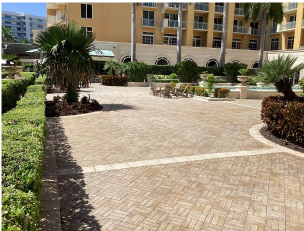
Plaza deck overview
