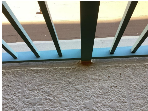
Railing post embedded in concrete
