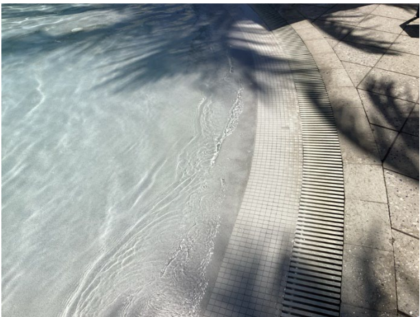
Pool plaster finish
