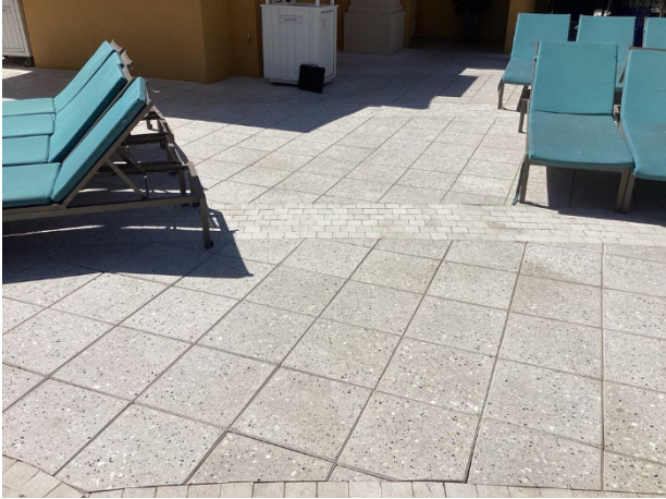
Paver pool deck overview
