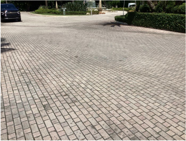
Masonry pavers at main entrance
