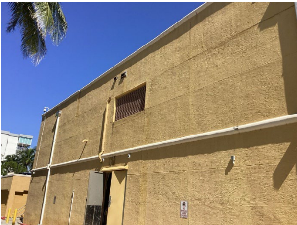
Stucco wall finishes
