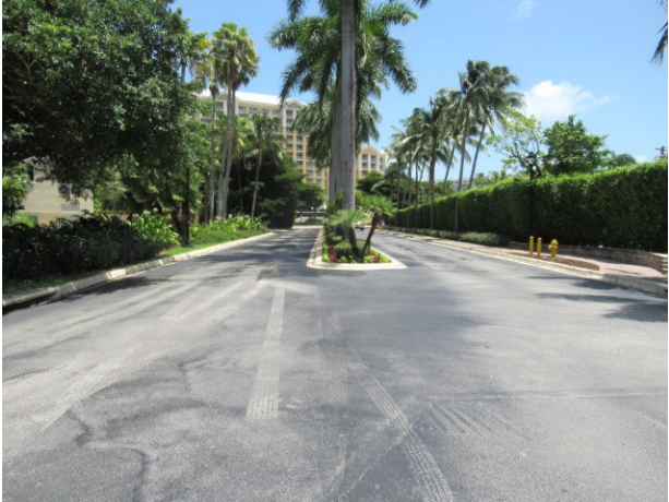
Asphalt pavement overview
