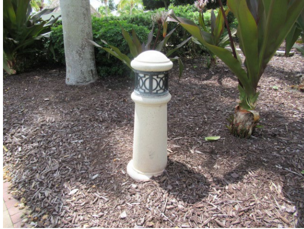
Bollard light fixture
