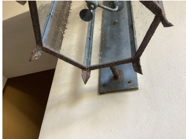
Finish deterioration
