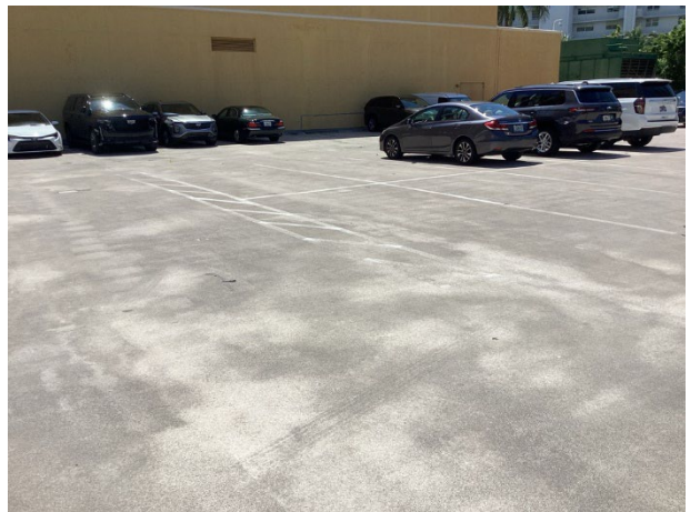
Elevated garage floor overview
