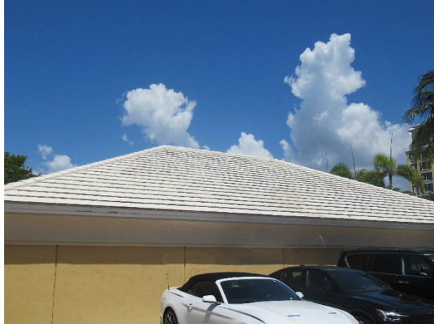
Concrete tile roof overview
