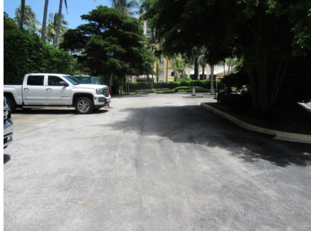
Asphalt pavement overview
