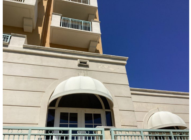
Finish deterioration
