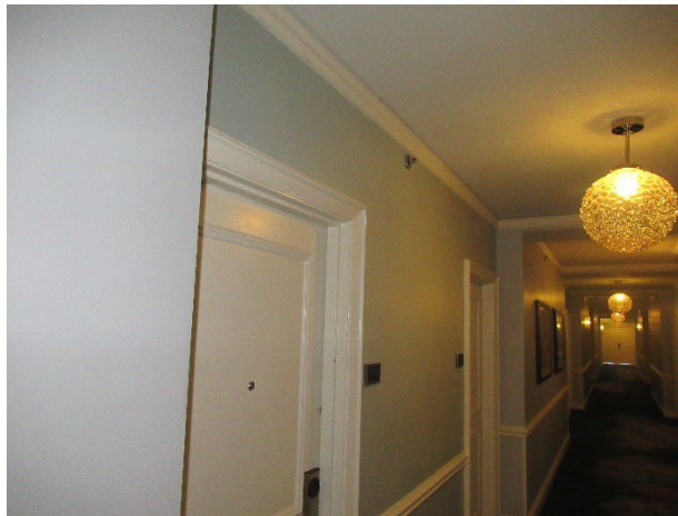
Hallway paint finishes
