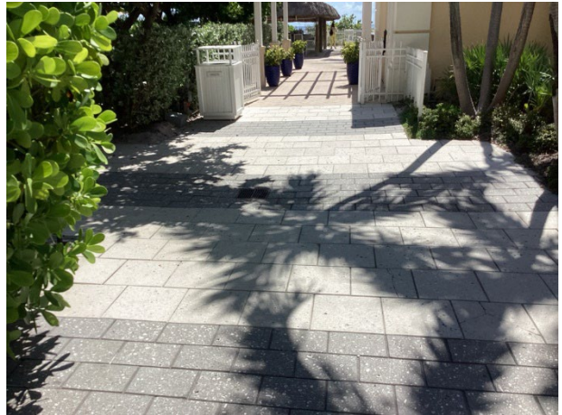
Paver pool deck overview
