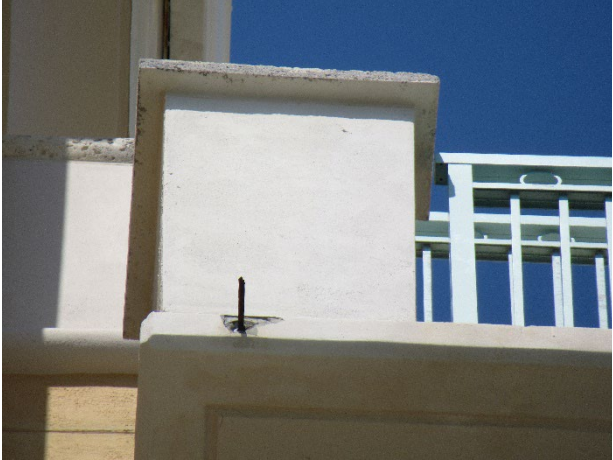
Exposed reinforcements
