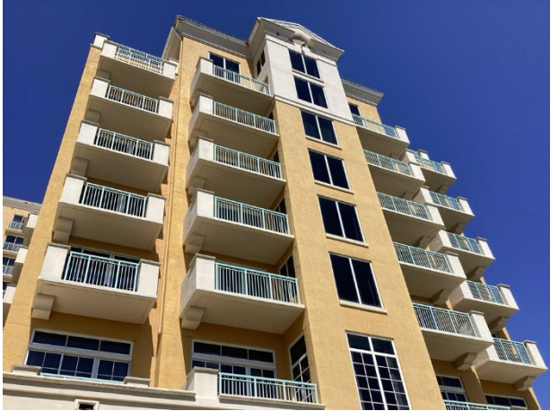
Stucco wall finishes
