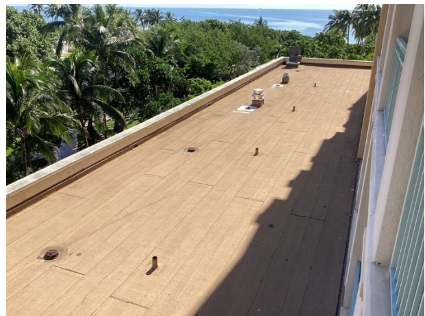
Flat roof overview
