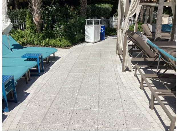
Paver pool deck overview
