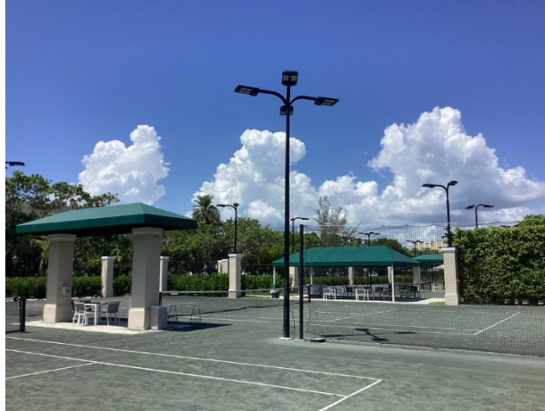
Sport court light poles and fixtures
