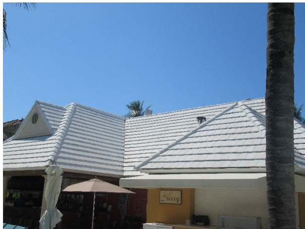
Concrete tile roof overview
