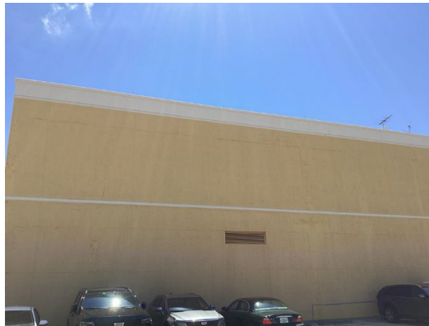
Stucco wall finishes
