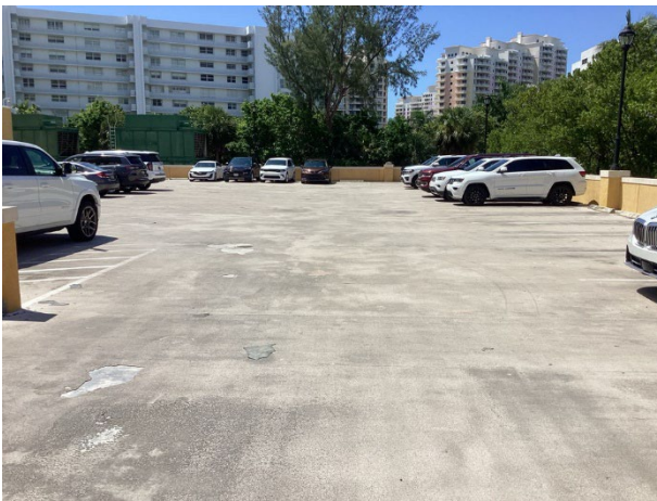
Traffic coating overview
