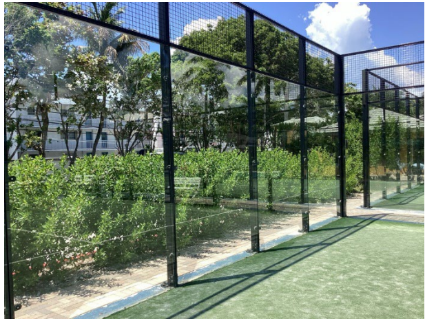
Padel court glass enclosure
