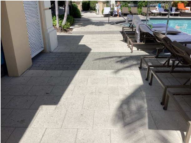
Paver pool deck overview
