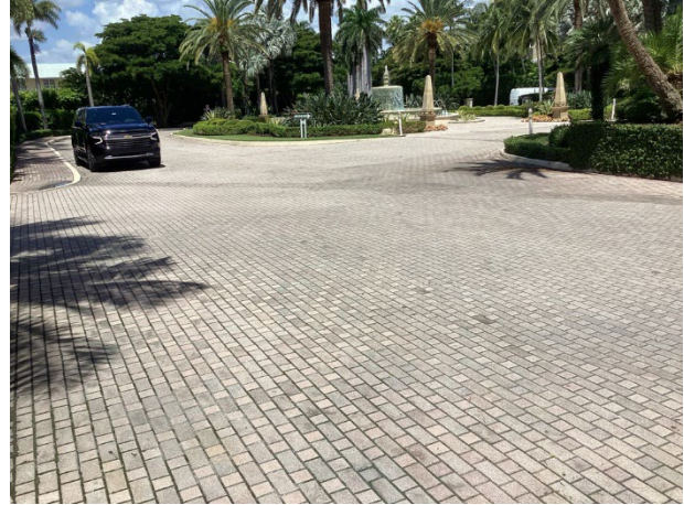
Area with underlying membrane overview
